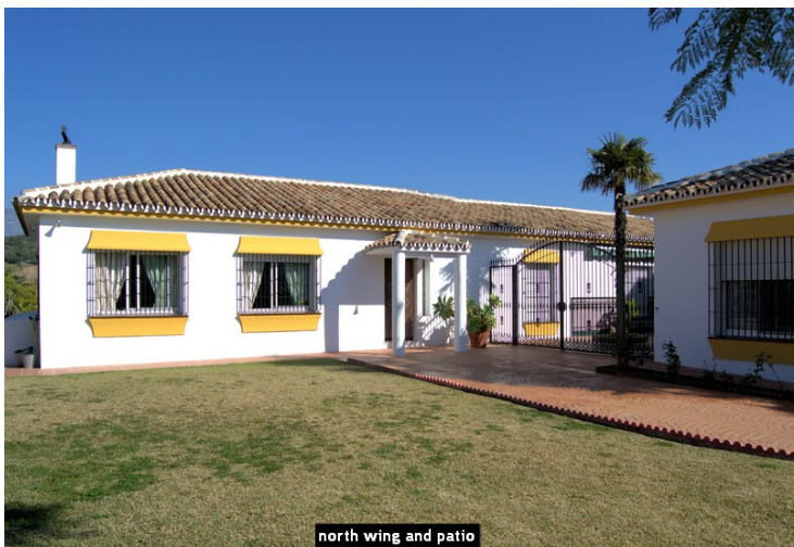
north wing and patio
