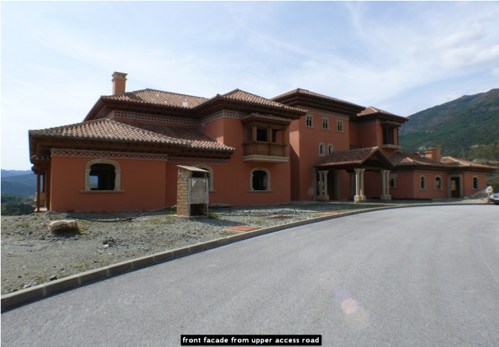
front facade from upper access road
